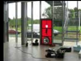
air tightness test
